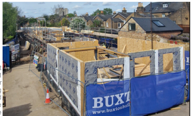
Plot No.1 Exterior being installed by the crane
