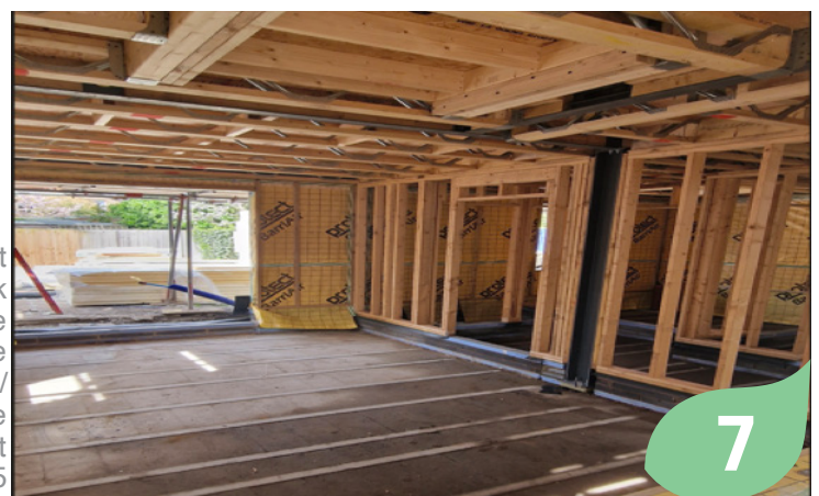
First look inside the Kitchen/Lounge of plot No.5
