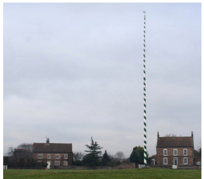
The maypole in Nun Monkton. Located on the extensive village green. Reputed to be the tallest maypole in England at 88 ft, and constructed in two sections, it replaced an earlier Norwegian Pine pole that collapsed during a gale in 2004. Photo © Chris Heaton (cc-by-sa/2.0)
