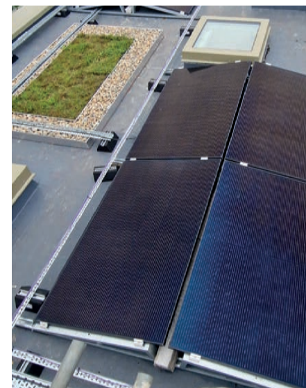
PVs, living roof and roof lights
