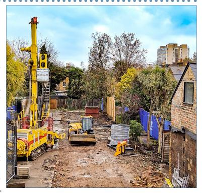
This meant that the expert had the task of carefully checking the boreholes during the drilling process using a magnet, every metre, for the first 10 metres of each hole.
